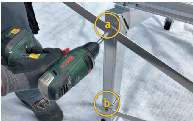
Figure 29: Position of drilled holes
