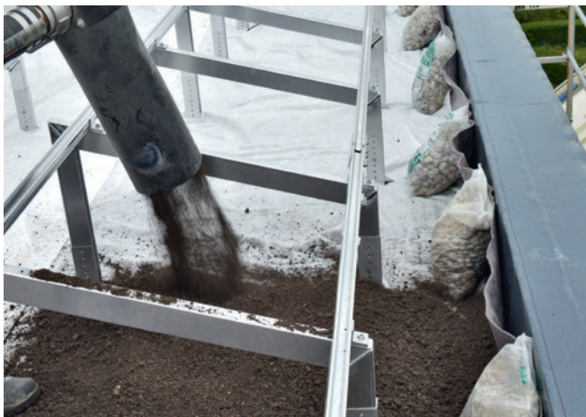
Figure 33: Blowing of the substrate.
