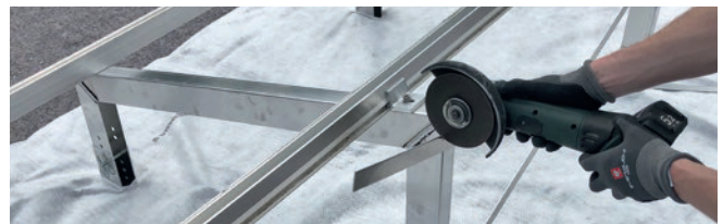
Figure 30: Cutting off the overhang from the wind bracing.
