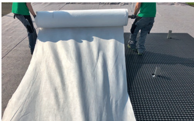
Figure 10: Rolling out the Filter Fleece.
