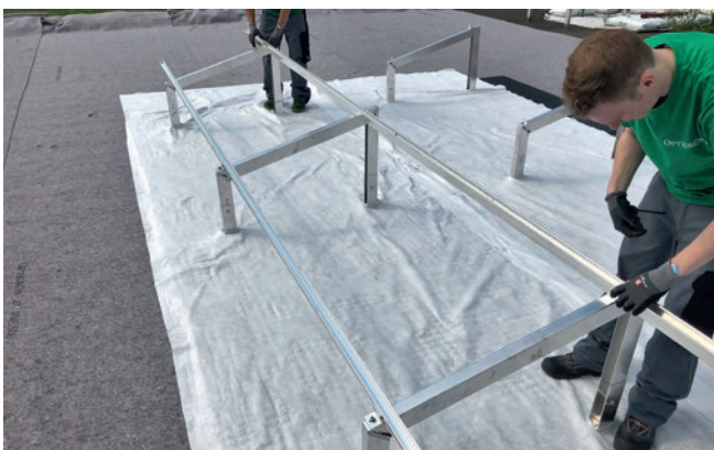
Figure 23: Mounting the second Easy Mounting Rail.
