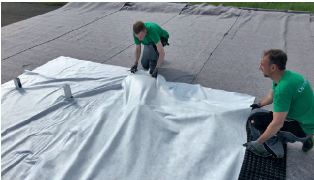
Figure 16: Lay second row of fleece.
