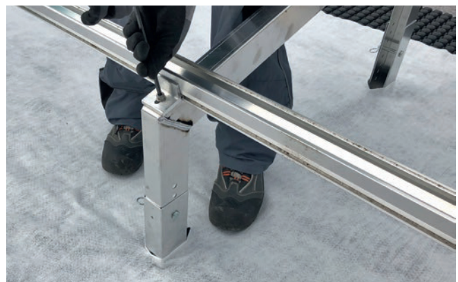
Figure 24: Tighten Rail Fixings.
