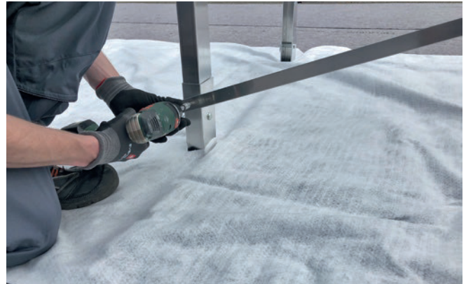
Figure 28: Fastening of the metal strip.
