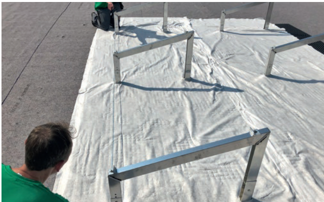
Figure 21: Alignment of the row using string
