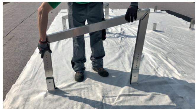
Figure 19: Mounting Frame on the Base Plate (example Mounting Frame).
